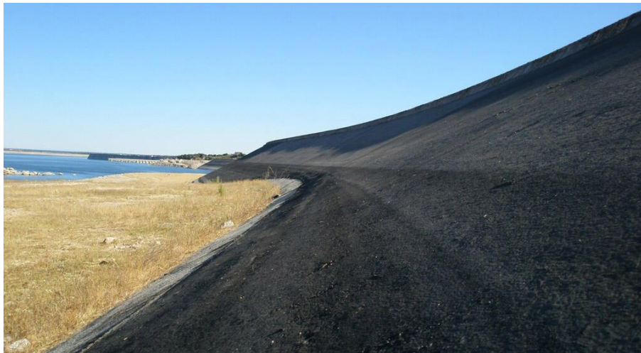
View of the dam showing the low water level (photograph: Perronaider)
