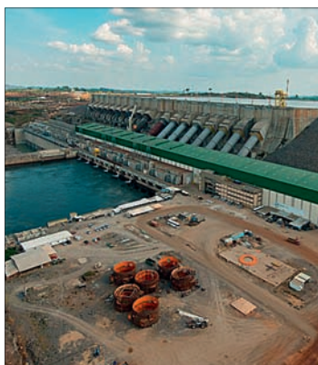
5. View of the Belo Monte powerhouse during construction.
