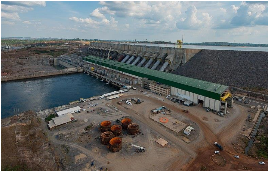
Belo Monte Hydropower Station (photograph: Fernanda Brandt )
